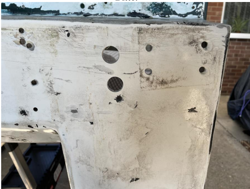
The holes for the heater pipes are adjacent to the left hand body to chassis brace.
